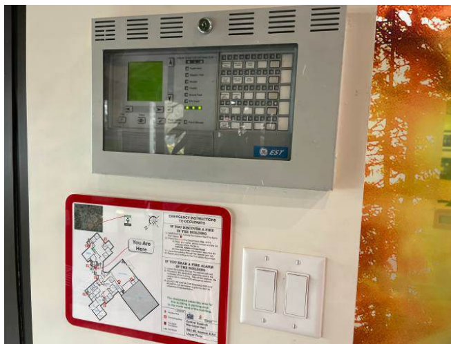
Photo #32: Fire Alarm Annunciator Panel
