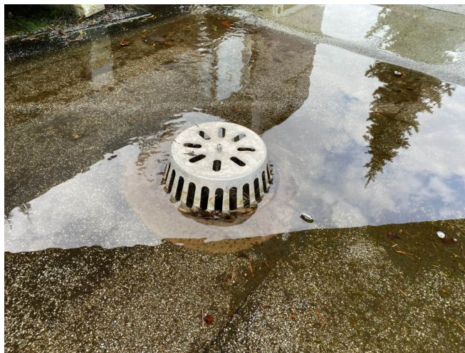
Photo #26: Flat Roofing - Ponding at Area Drain
