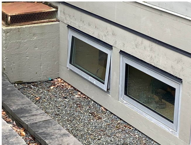
Photo #12: Windows-Newer Aluminum Awning - Typical
