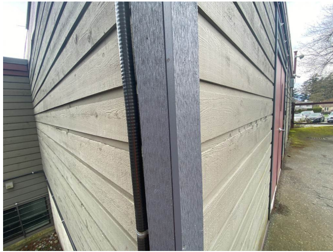
Photo #5: Cladding- Wood Trims at Corners - Typical
