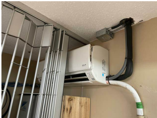
Photo #39: HVAC - Split System Unit- Typical
