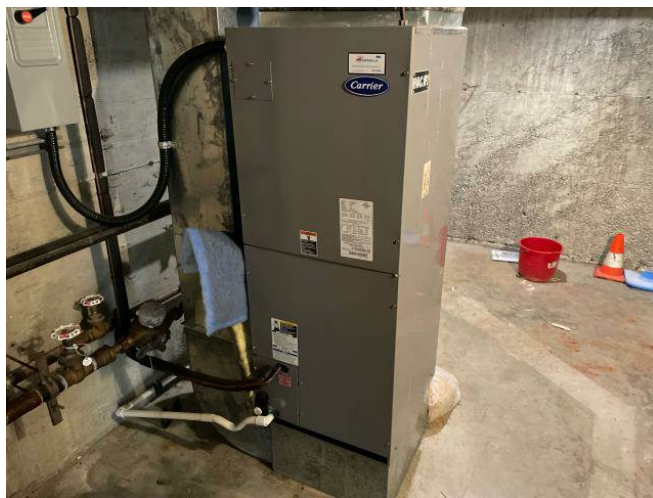
Photo #41: HVAC - Furnace
