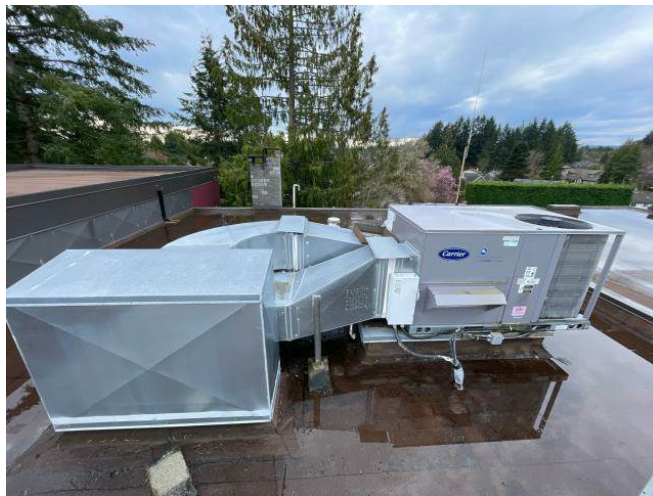
Photo #38: HVAC - Rooftop HP Package Unit- Typical2
