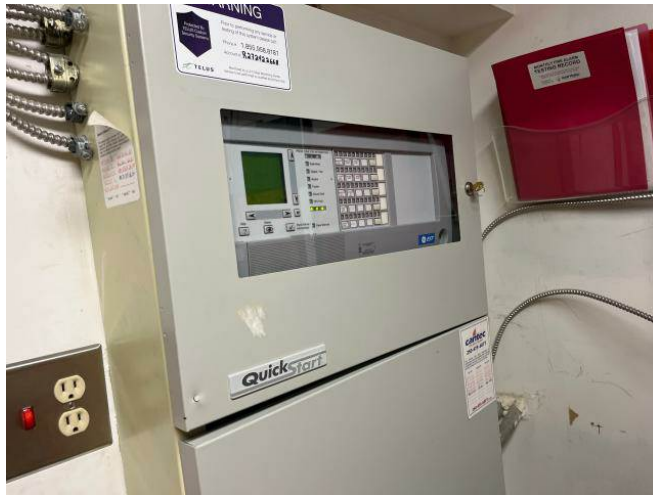
Photo #31: Fire Alarm Panel
