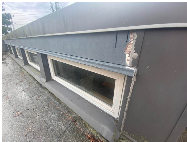
Photo #8: Cladding Failure- Municipal Clerestory
