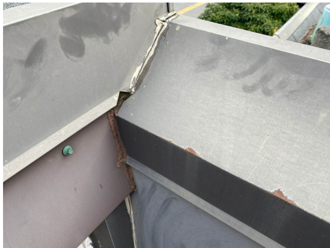
Photo #27: Parapet Metal Flashing- Sealant Failure
