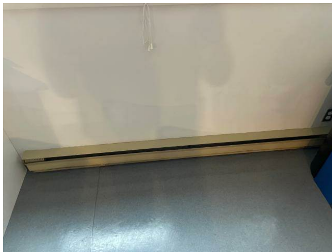
Photo #44: HVAC - Electric Baseboard Heater
