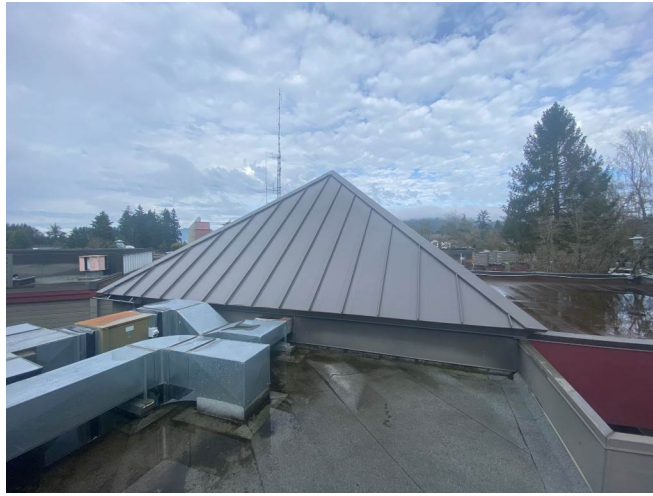
Photo #28: Roofing- Sheet Metal Dome
