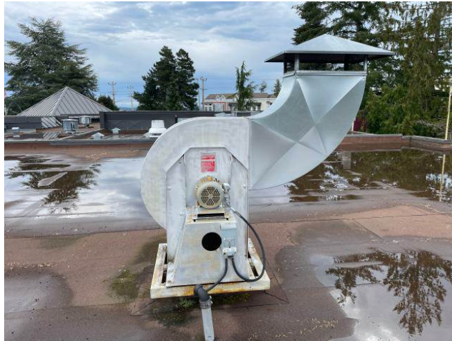
Photo #43: HVAC - Fire Department Apparatus Bay Exhaust Fan
