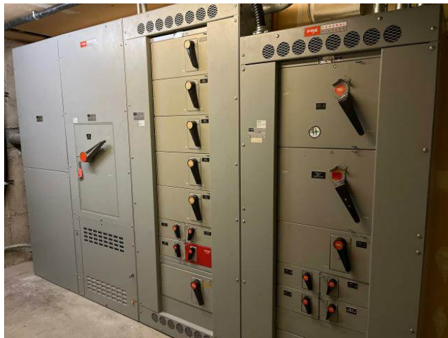
Photo #48: Electrical Main Switchgear
