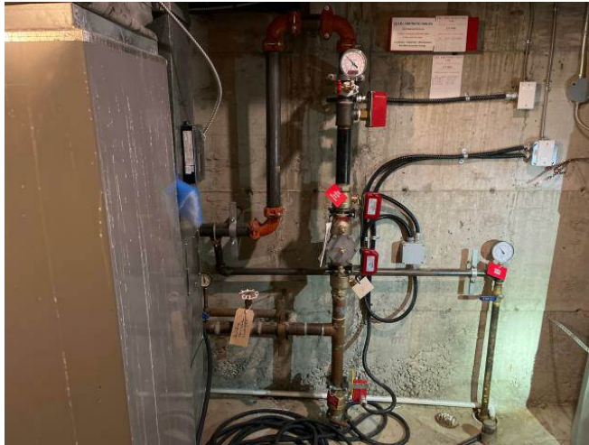
Photo #34: Fire Sprinkler Riser
