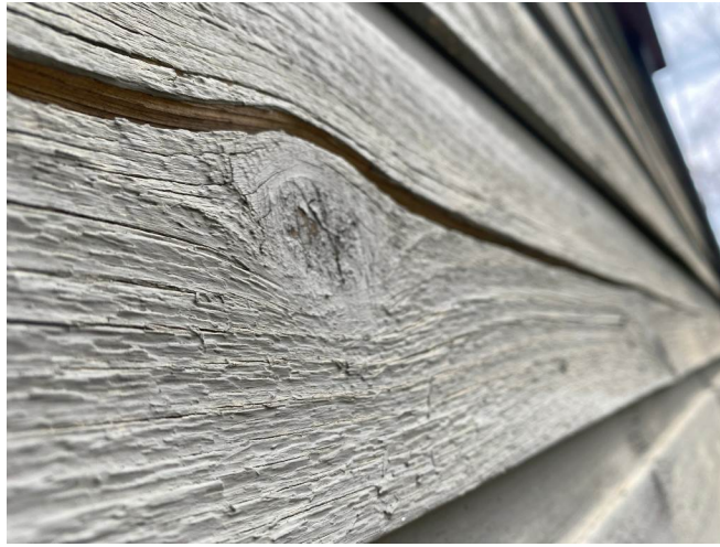
Photo #7: Cladding-Wood Siding - Southeast Weathered
