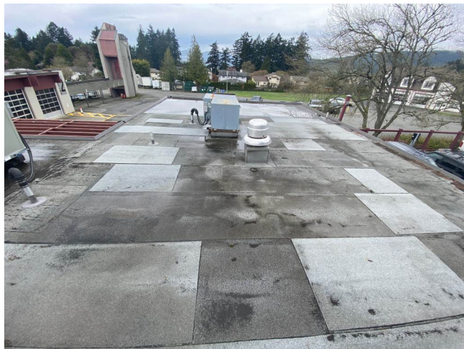
Photo #24: Flat Roofing in Poor Condition - Typical
