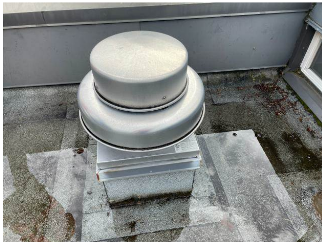
Photo #42: HVAC - Rooftop Exhaust Fan - Typical
