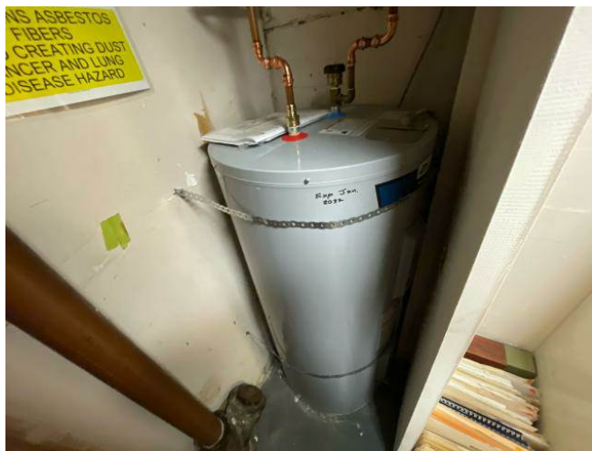
Photo #47: Domestic Hot Water Tank - Typical
