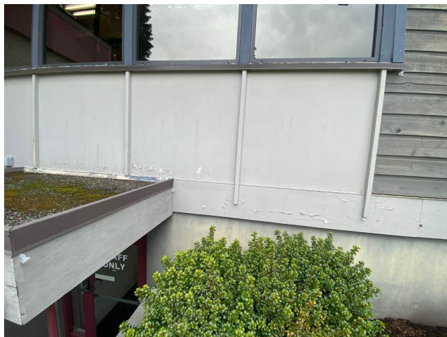
Photo #9: Cladding - Crezon Plywood with Peeling Paint
