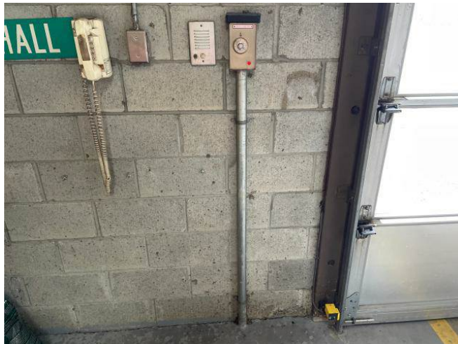
Photo #45: HVAC - Firehall In-Floor Heating Control
