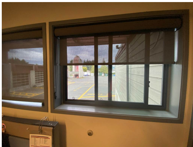
Photo #11: Windows- Double Glazed Aluminum - Typical
