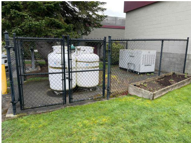
Photo #36: Generator- Propane (Outdoor)
