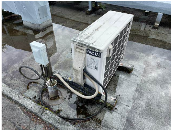
Photo #40: HVAC - Split System HP- Condenser - Typical
