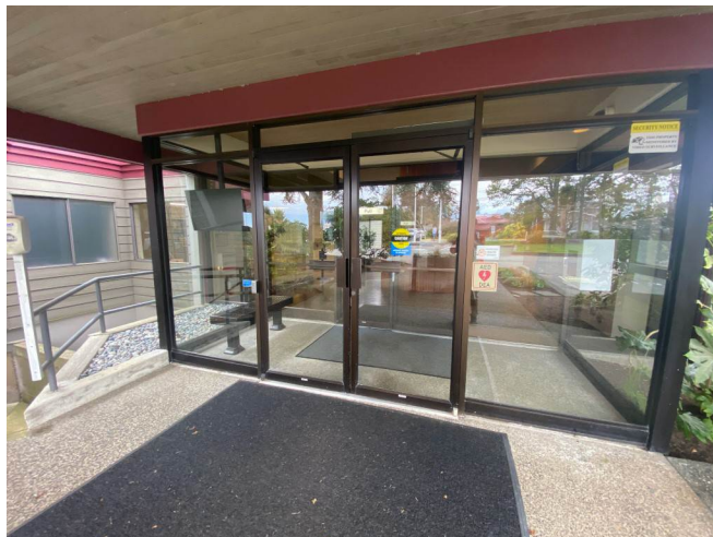
Photo #15: Exterior Door- Aluminum - Main Entrance
