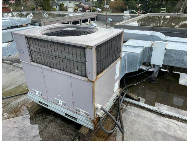
Photo #37: HVAC - Rooftop HP Package Unit- Typical1
