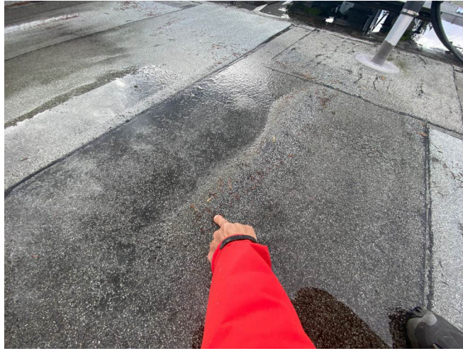
Photo #25: Flat Roofing Blister and Alligator Cracks
